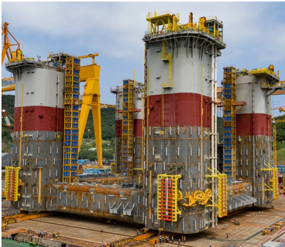
Fig. 1 FPU hull constructed by Hanwha Ocean
